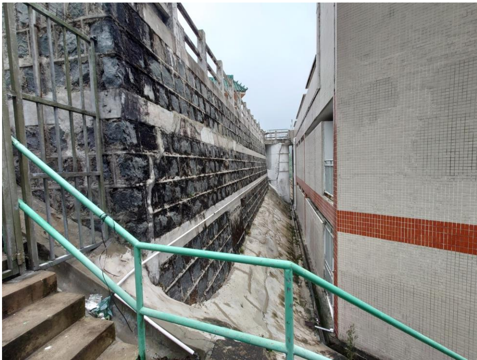
Photo L – General View of the Feature No. 11SE-D/CR341
