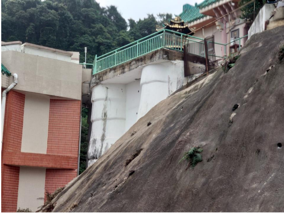
Photo K – General View of the Feature No. 11SE-D/R63
